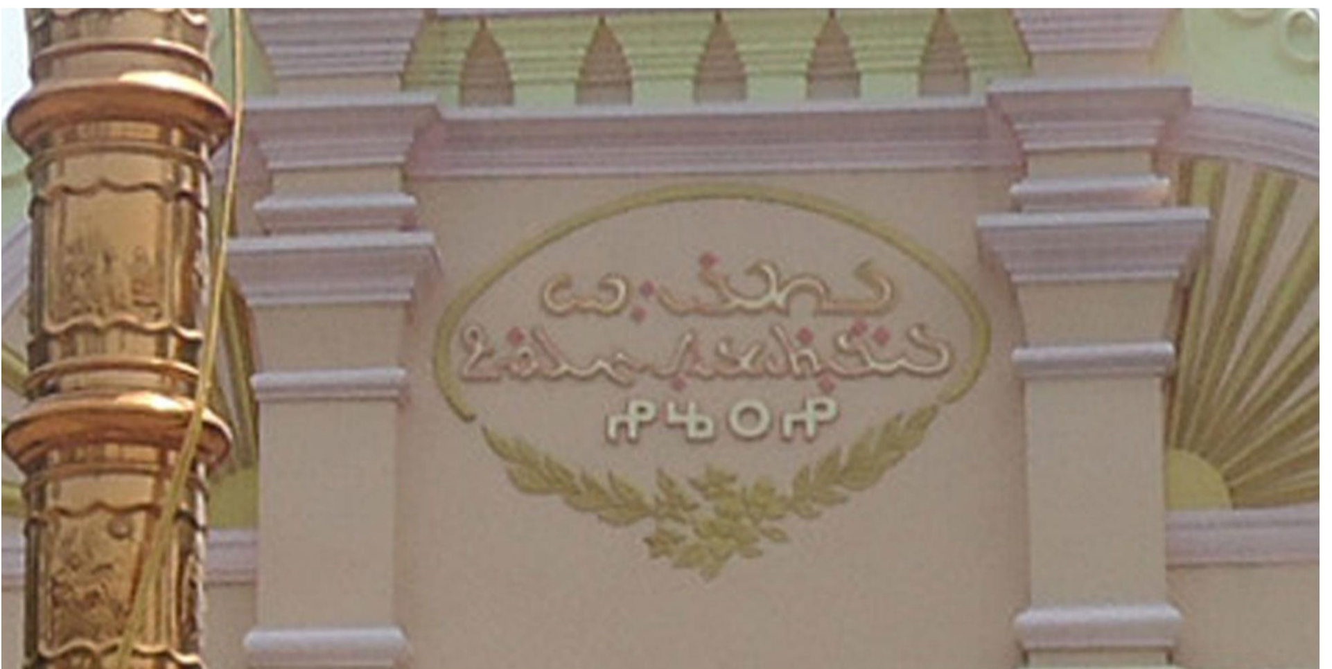
The façade with Syriac inscriptions at Holy Cross forane Church, Manjapara
